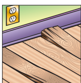
▲ loose floorboards
